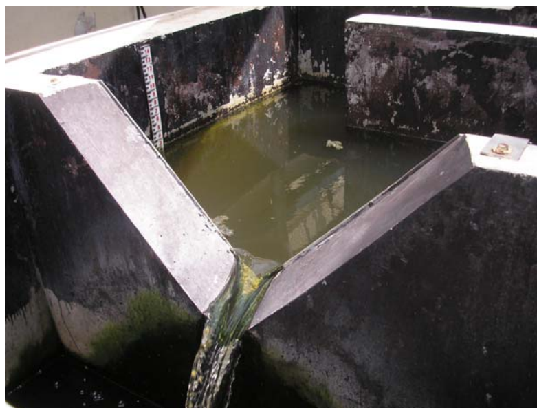
Figure 6.8 Sample Collection from a V-Weir
