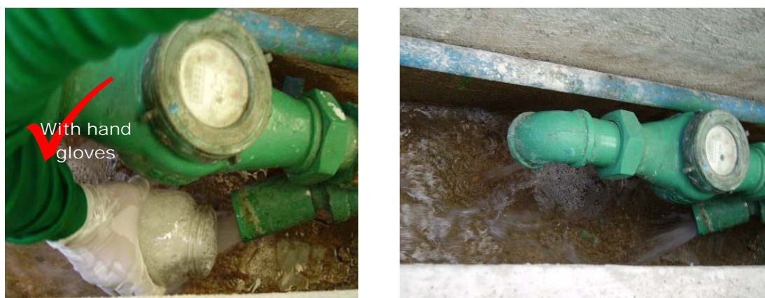
Figure 6.10 Direct Sampling using sample container, at specified sampling station
